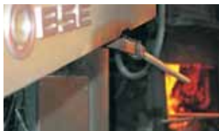
In and out through the slag door – without any process interruption!
